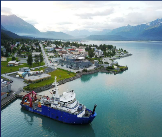
Seward Marine Center Dock Replacement
